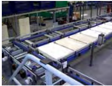
Figure 9. EBS elements, here storing a line of empty totes
